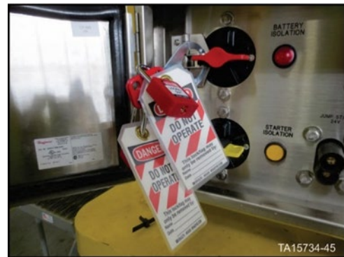
Figure 33. Battery Isolation Box – Battery isolation switch in OFF position with locks in place
