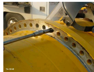
Cleaning paint and rust prior to torquing
